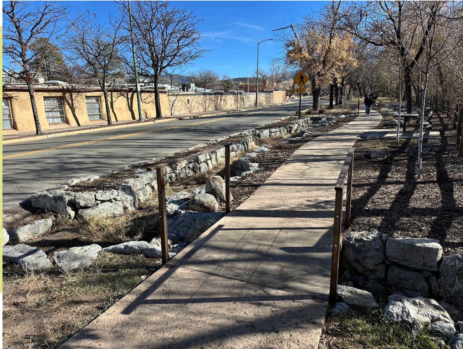
Green Stormwater Infrastructure
