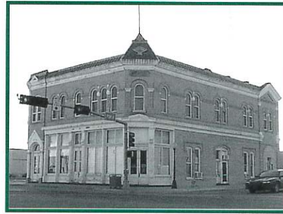
The landmark Carlsbad Irrigation District Building has garnered the community's interest for redevelopment and rehabilitation
