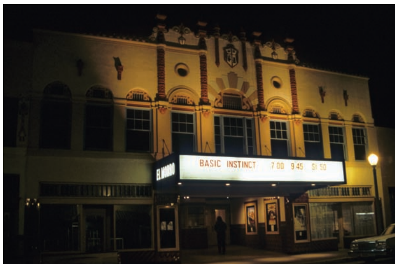
LEFT TO RIGHT: TOP LEFT El Morro Theater rehabilitation, Gallup, ca. 1991. Photograph by Elmo Baca, NMMS. TOP MIDDLE El Morro Theater rehabilitation, Gallup, ca. 1991. Photograph by Elmo Baca, NMMS. BOTTOM LEFT El Morro Theater after rehabilitation, Gallup, ca. 1992. Photograph by Elmo Baca, NMMS. RIGHT Artist's gallery and studio, Raton, 2010. Photograph by Elmo Baca, NMMS.
