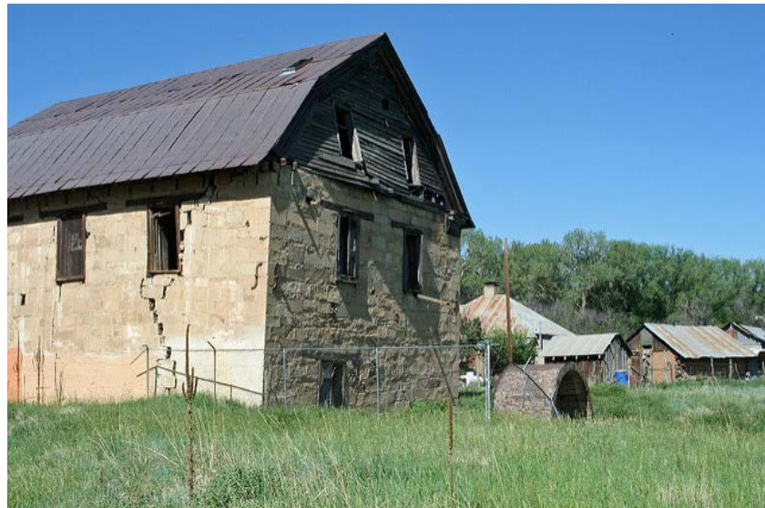
Historic St. Vrain Mill, Mora
